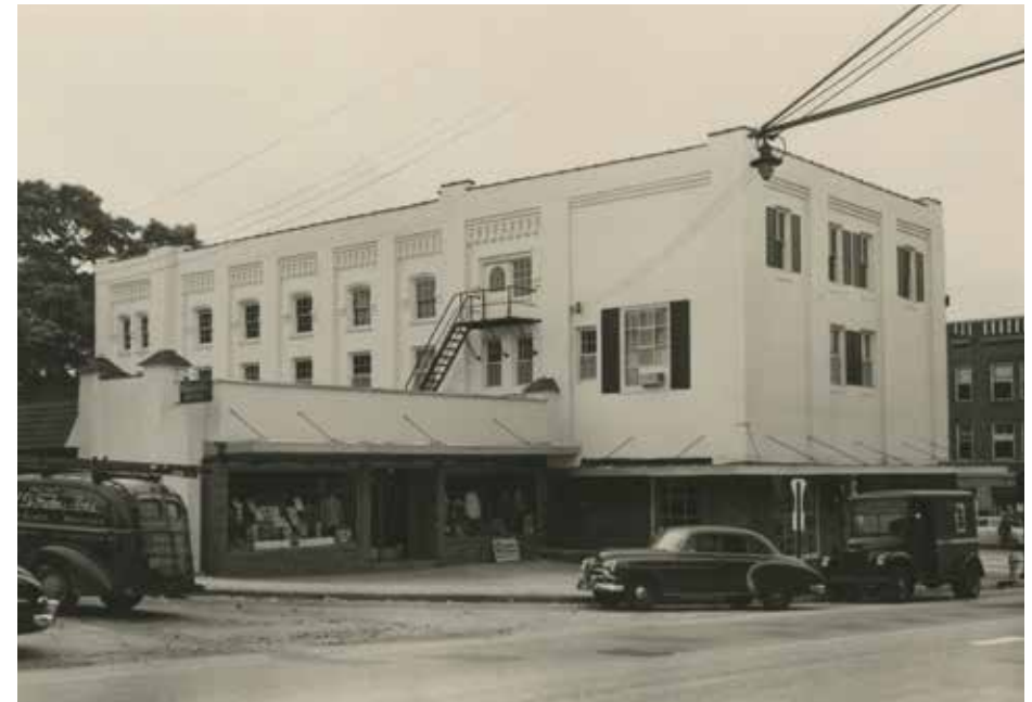
Above: The completed renovation simplified the building's exterior but added elements like false shutters. Below: On the north facade, less was changed. The original ornamental arches over the windows were retained, and can still be seen today. A flat roof cantilevering over the sidewalk provided shade to the stores.
