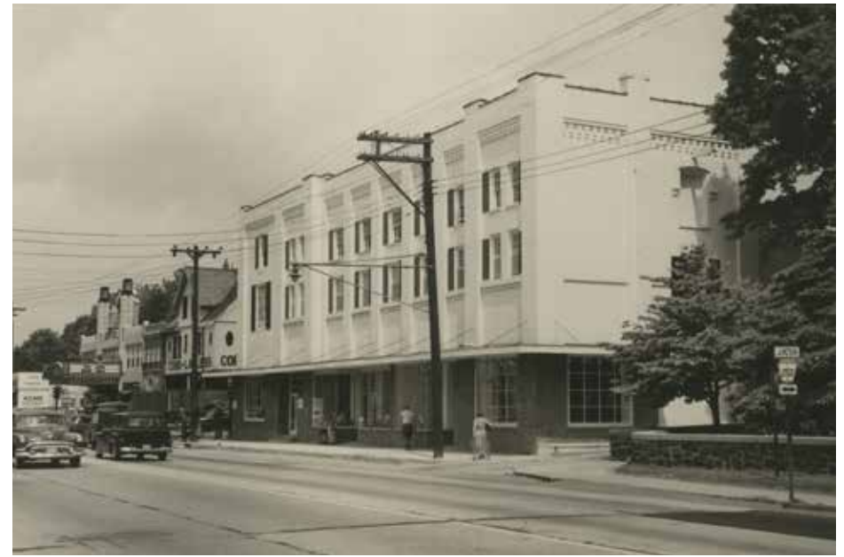
Above: The completed renovation simplified the building's exterior but added elements like false shutters. Below: On the north facade, less was changed. The original ornamental arches over the windows were retained, and can still be seen today. A flat roof cantilevering over the sidewalk provided shade to the stores.
