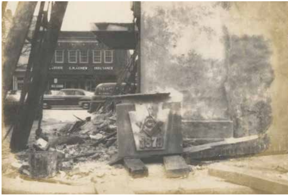
Above: The building's datestone, bearing the Masonic emblem and "1871" construction date, was removed during the renovation. Below: This interior view of the third floor before partitioning for new offices provides once last look at the once open theater space that also included the floor below.
