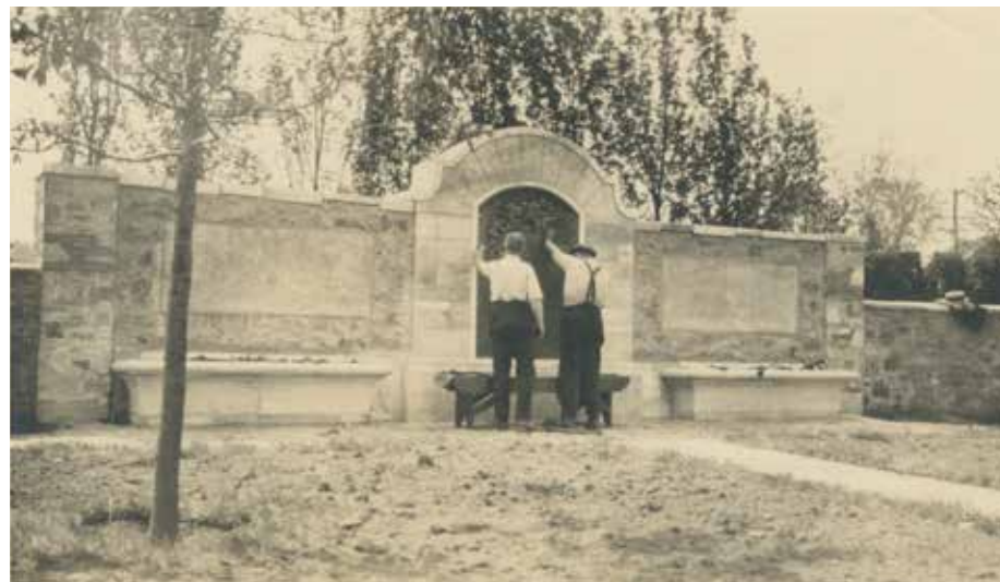
The finished bronze tablet being set into the memorial wall.
